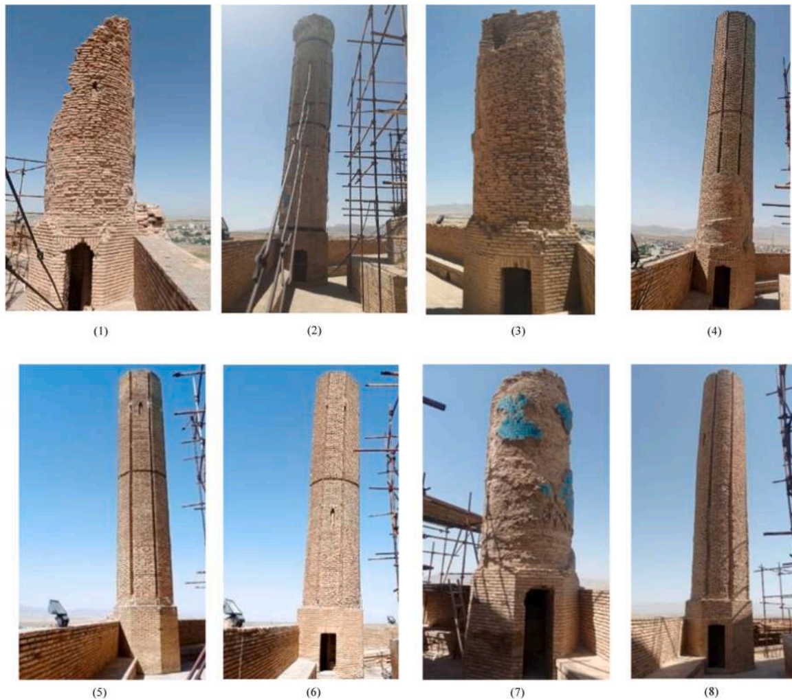
Fig. 11. Global conservation works and structural retrofitting of the eight minarets.
